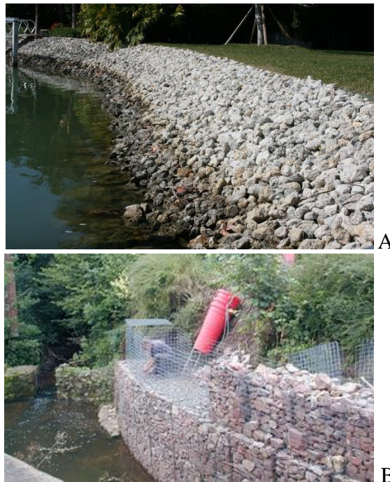
Figure 1 : Riprap (A) and Gabion (B)
