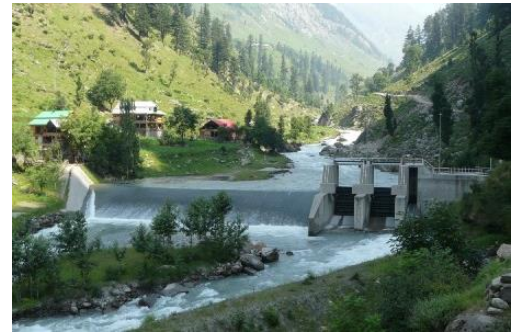
Photo- Example of ROR dam
