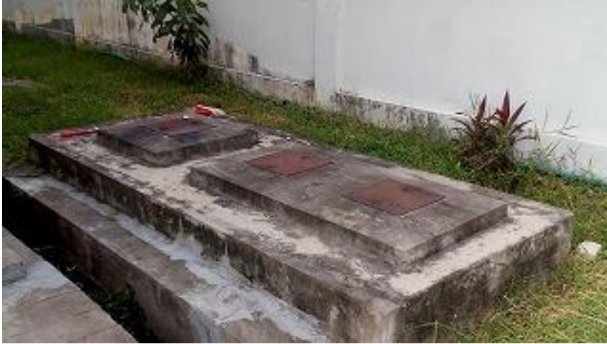
Figure: Common Septic Tank
