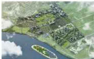
Dagon Seikkan Smart District 1,000 acres of urban infrastructure development and 300 acres of land for private and commercial development
