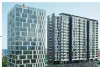
Crystal Tower and Crystal Residences 1.2 million sqft of integrated development, including 159 residential units in Crystal Residences
