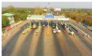
Sagaing Highway 188 km of toll road connecting 3 major cities in Upper Myanmar
